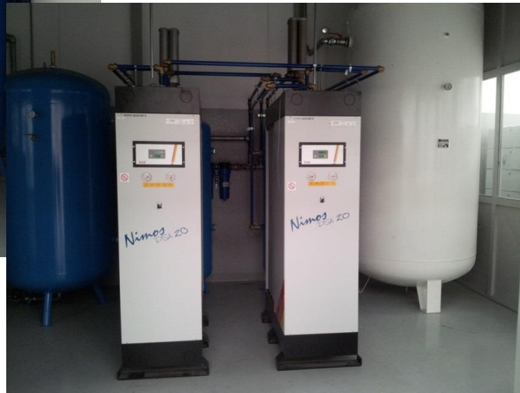
N. 2 PSA SL2 -20 – 2 x 33,9 m 3 /h Purity 99,5% - Caffè Vergnano – Santena - ITALY Food Industry- Coffee
